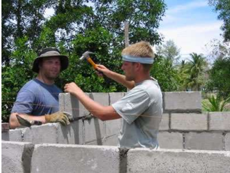
Wave of Hope volunteers crafting the trade of brick laying at Tap Tawan Village.
